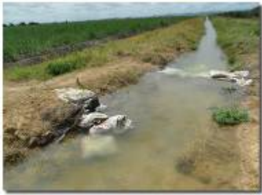
Not ideal: Makeshift control structures in Manyonyo
