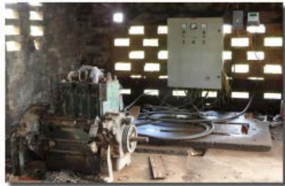
Old and new: the old diesel pump at Buleya replaced with an electrical one.
