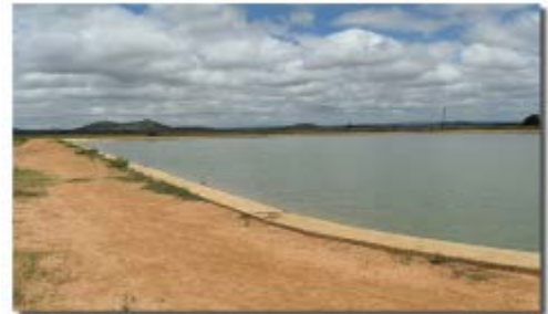
A well constructed reservoir at Manyonyo, but with an outlet that might be too small
