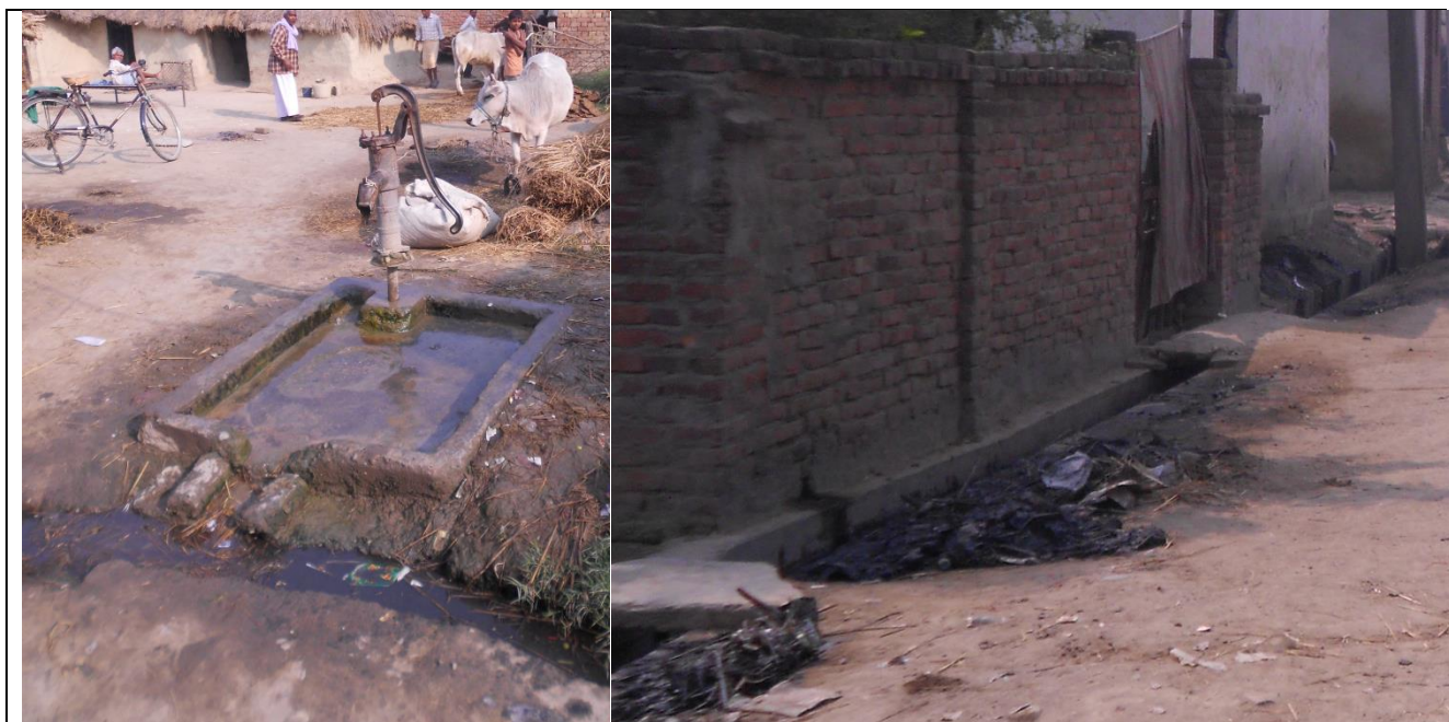
Figure 5 Drainage problems in Terai
